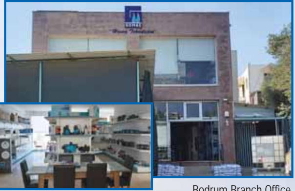
Bodrum Branch Office
